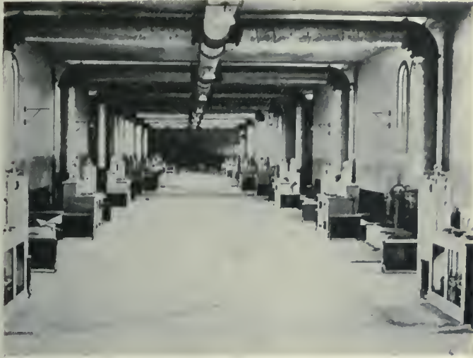
Fig. 6—Completed Prefilter Gallery.
